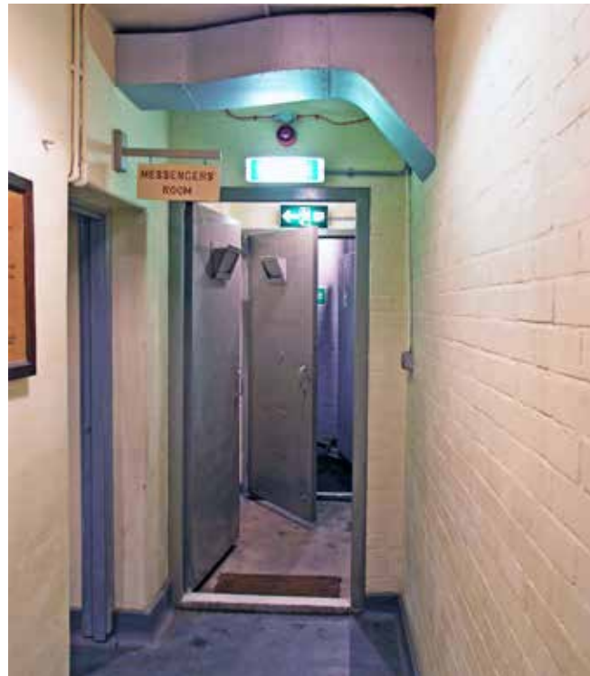
Spine corridor looking back towards the entrance doors, with their flapped apertures. Photo Victor Smith
